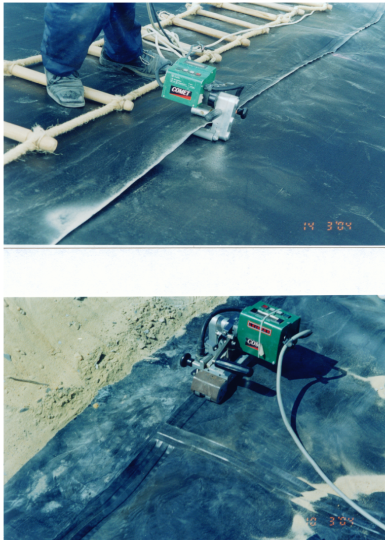
Welding with Hot Wedge Fusion Machine
